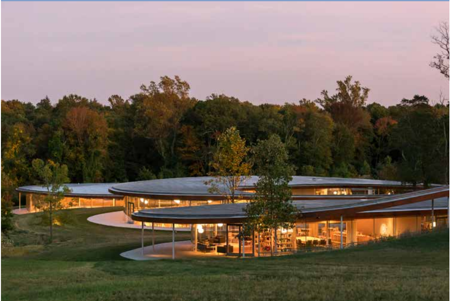
Designed by SANAA, the River building was created as a porous platform for the work of Grace Farms Foundation. Structurally, the building of glass, concrete, steel, and wood is in essence a single long roof, which seems to float above the surface of the ground as it twists and turns across the landscape. (Photo: Dean Kaufman)
